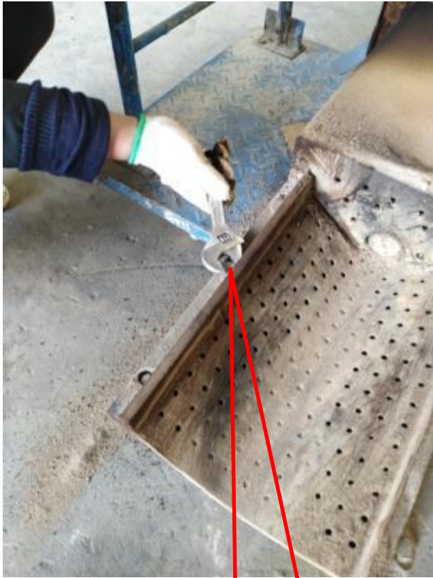
拆除固定螺栓
