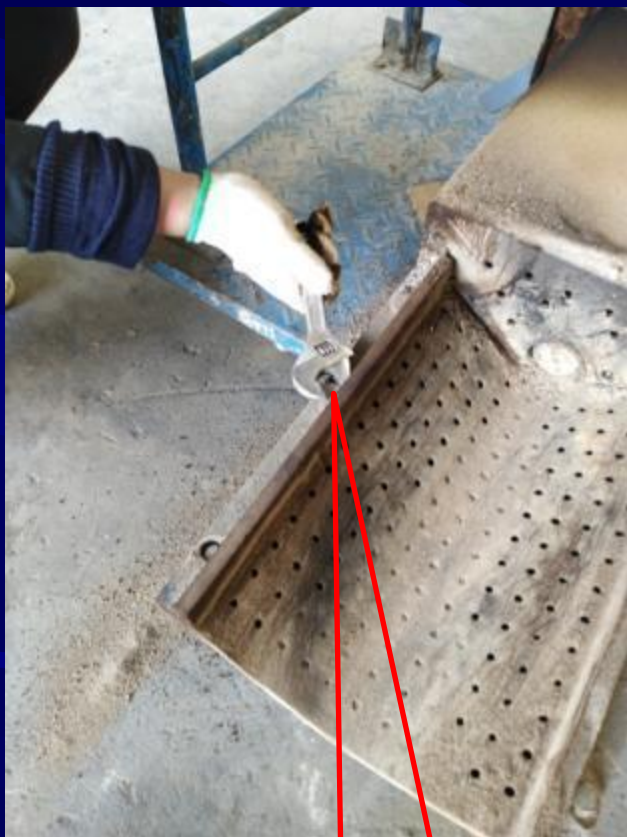
拆除固定螺栓
